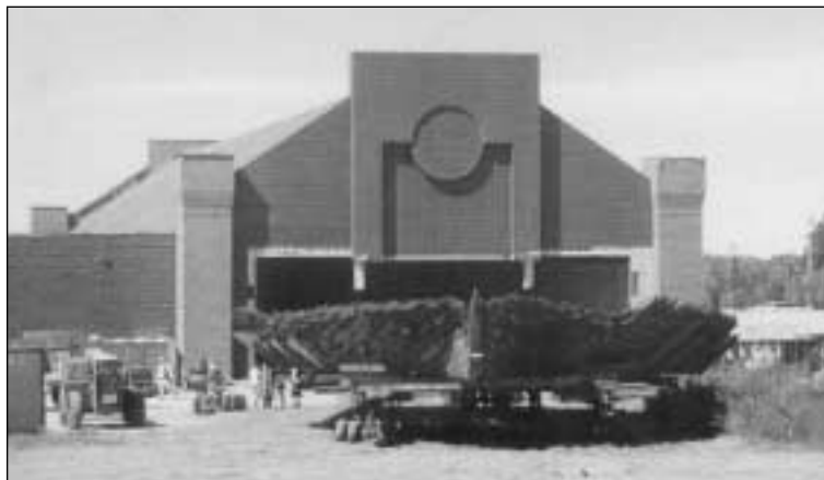
A big hurdle was passed in early October when the remains of the CSS Jackson were moved into the new museum building. The end of the building was left open to allow placement of the ship, which was 180 feet long.
