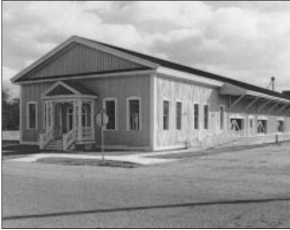
Eufaula/Barbour County Chamber of Commerce to be housed in the newly renovated Central of Georgia Depot
